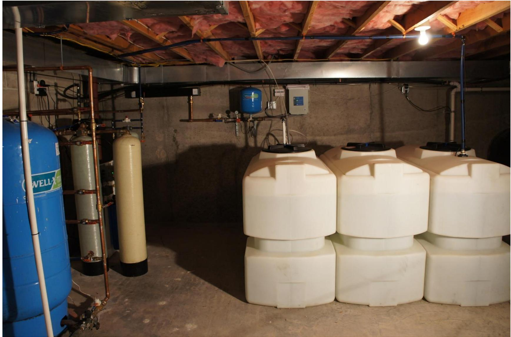
The RO water will flow through a tank filled with crushed limestone before going in to the storage tanks. This will add some minerals back to the water and raise the PH.
