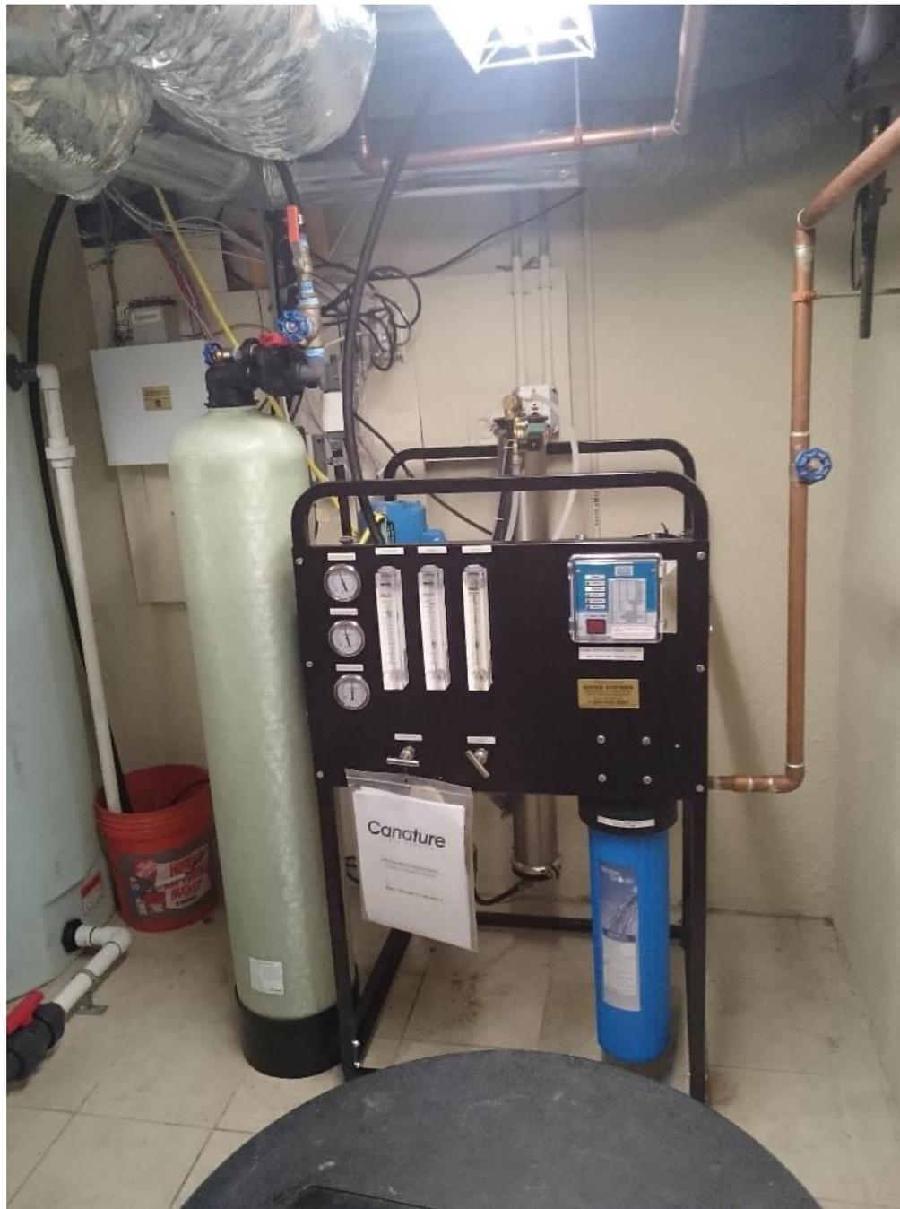
This is using an alternating water softener as pretreatment for hardness. It regenerates based on water use. One unit is on line at all times.
