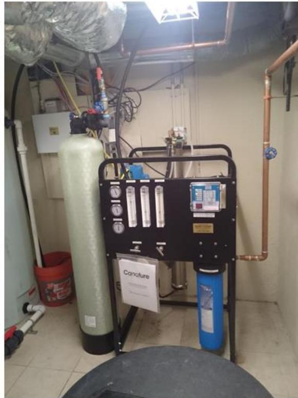
This is a external booster pump drawing the water out of the tanks and sending it in to the house.
